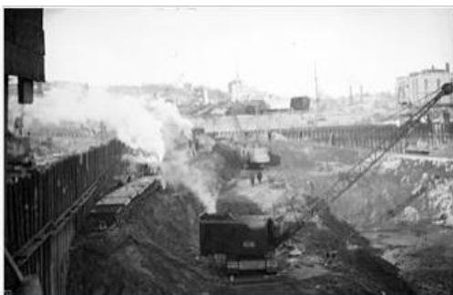
Construction of the bunker
