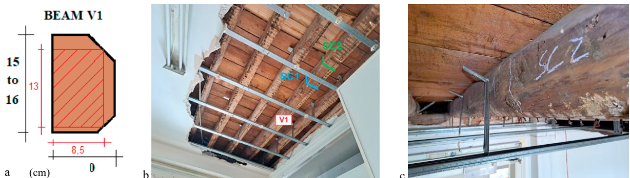
Fig. 2. (a) Beam cross-section; (b) The floor and beam V1 with critical cross-sections; (c) Beam V1 in the zone of critical cross-section 2.
